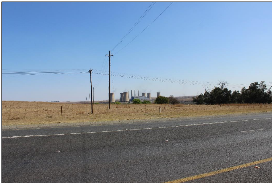
Figure 19: View of Camden Power Station to the west of the N2 national route.
