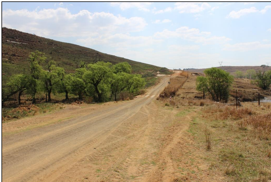
Figure 7: Areas of greater relief along the Vaal River to the south of the Camden 1 SEF project area.
