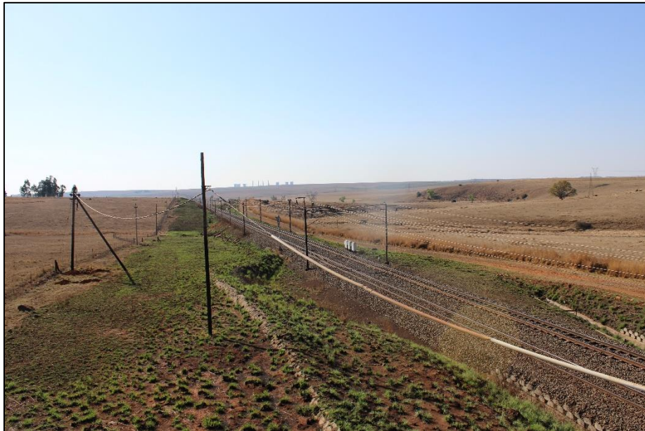
Figure 21: Rail infrastructure and power lines to the south-east of the Camden 1 SEF project area.
