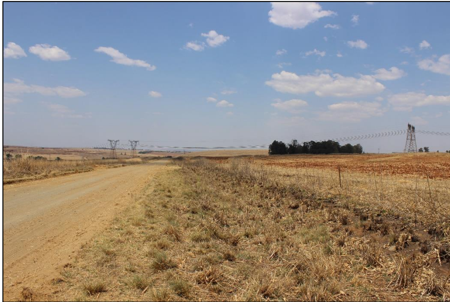
Figure 20: High voltage power lines feeding into Camden Power Station.
