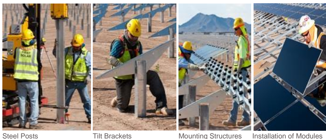
Figure 4: Fixed tilted mounting structure for PV Array (Web 4)
