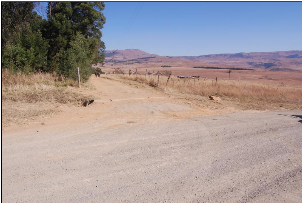
Plate 2 POI2 – D699 / Site Access Track Intersection
