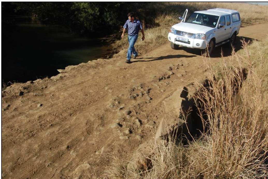
Plate 1 POI1 – Site Access Track Crossing of Stream
