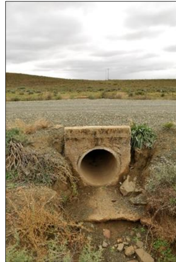
Plate 2: existing pipe culvert
