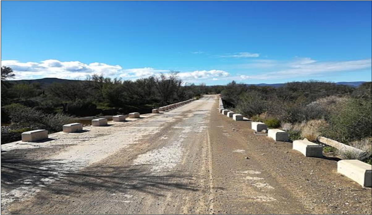
Figure 51: Narrow bridge on DR02249
