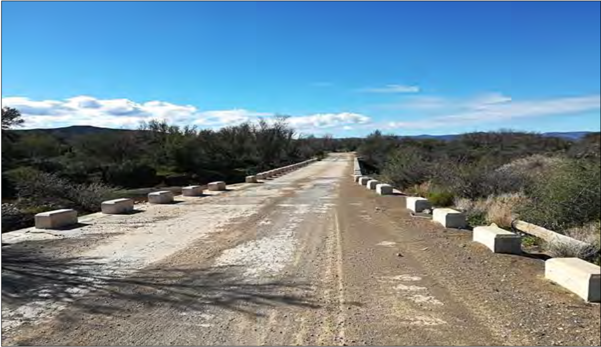
Figure 38: Narrow bridge on DR02249
