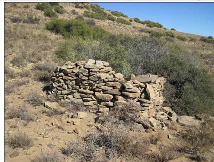
View of stone packed wall at site UMS007
