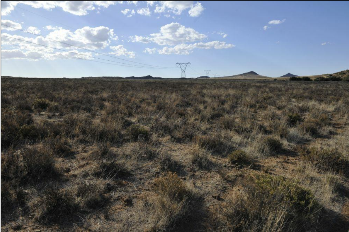
Figure 29: Hydra-Poseidon 400kV 1 high voltage line running through the study area
