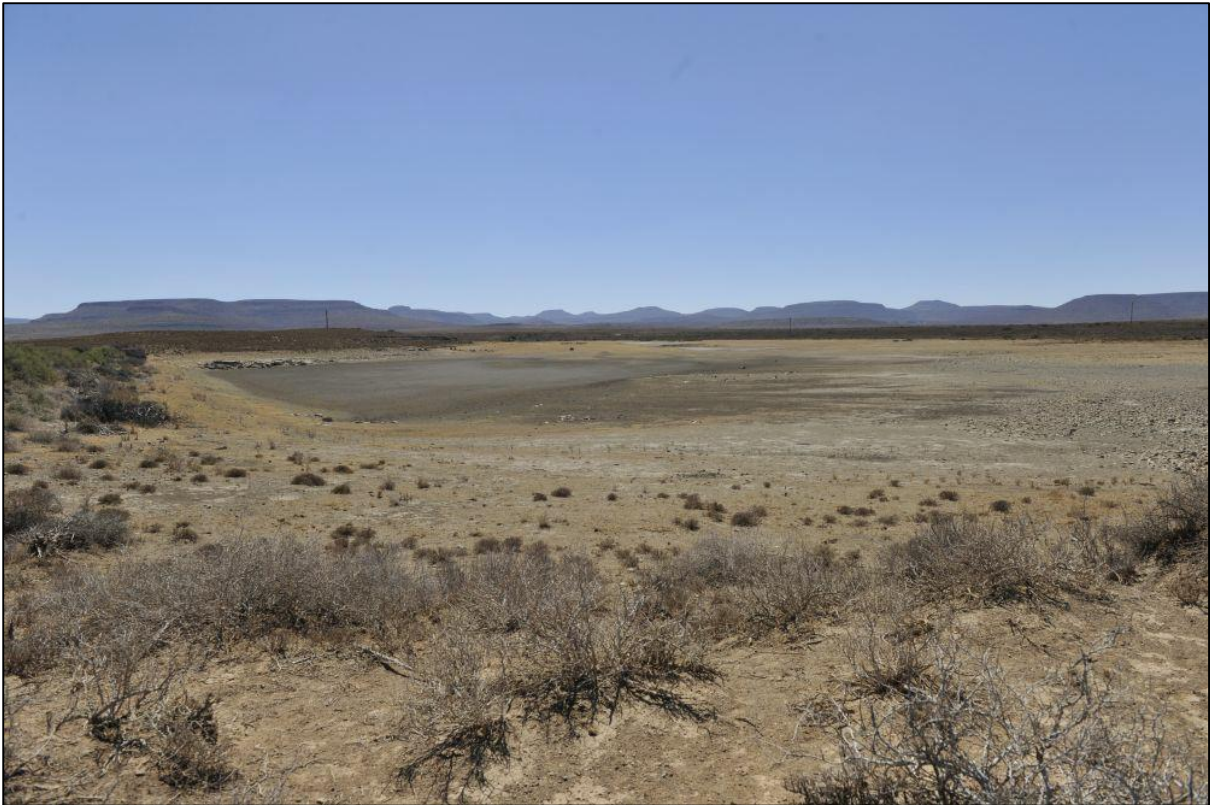
Figure 27: A dam in study area
