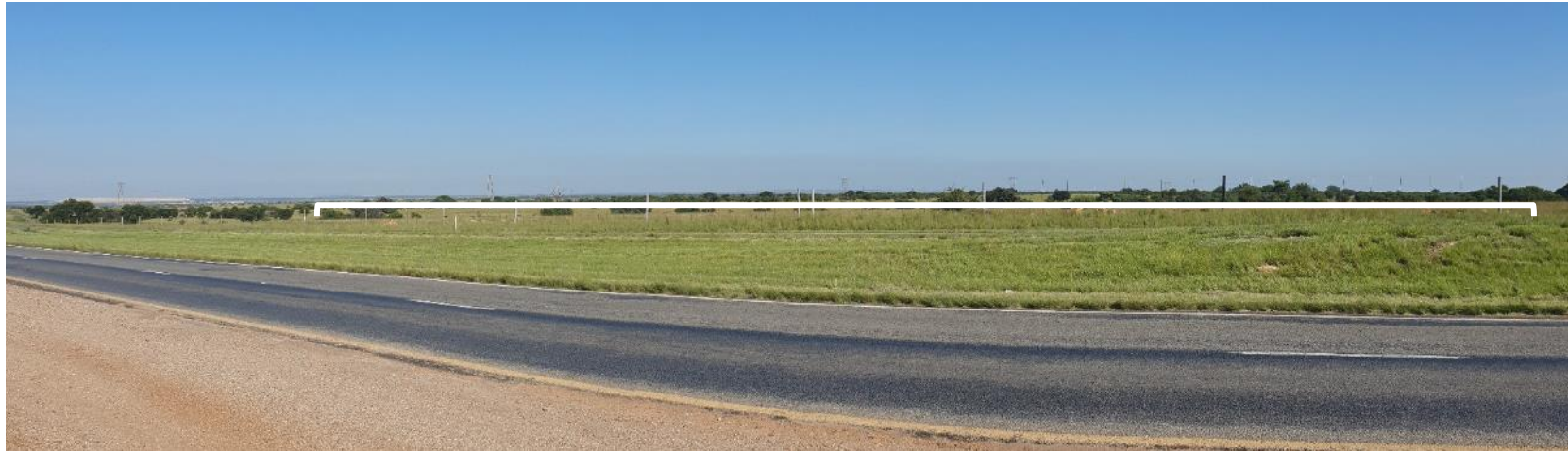
Viewpoint 5 (N12) looking north towards the Stilfontein PV Cluster in the middleground
