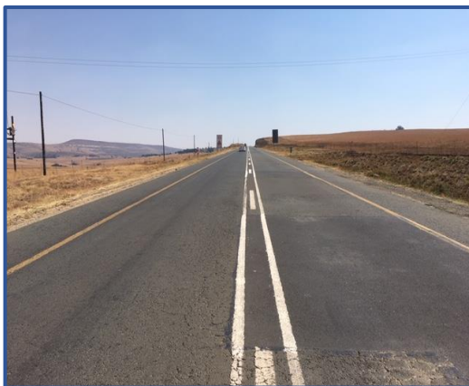
N2 Freeway – Looking west.
