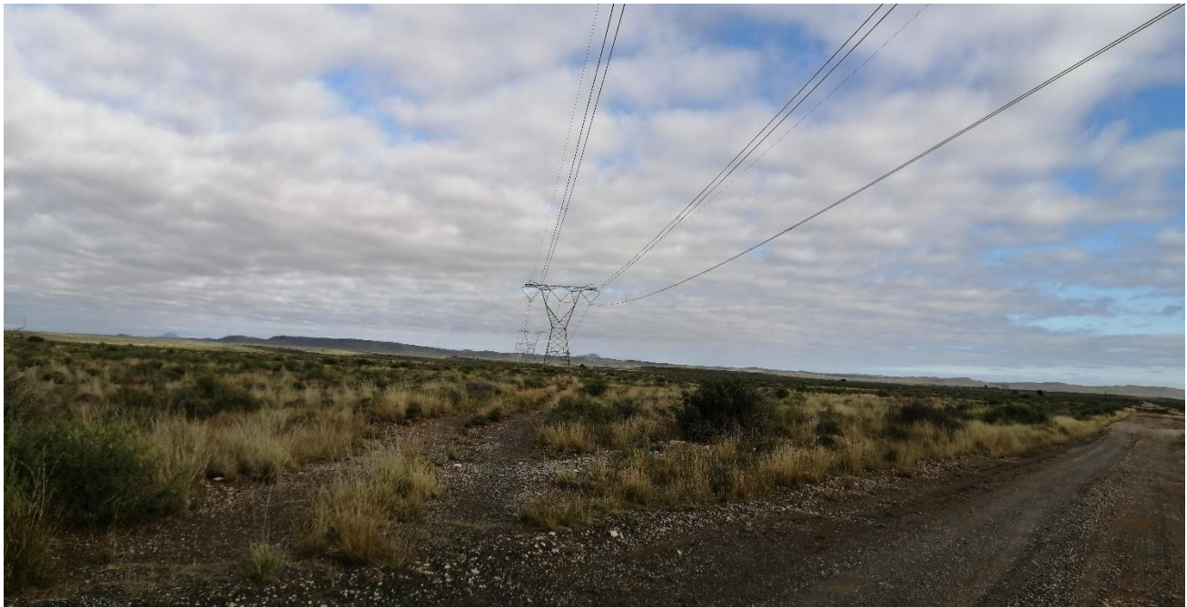
Figure 8: Existing powerlines in the study area
