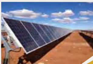
Bui solar photovoltaic (PV) feasibility study
