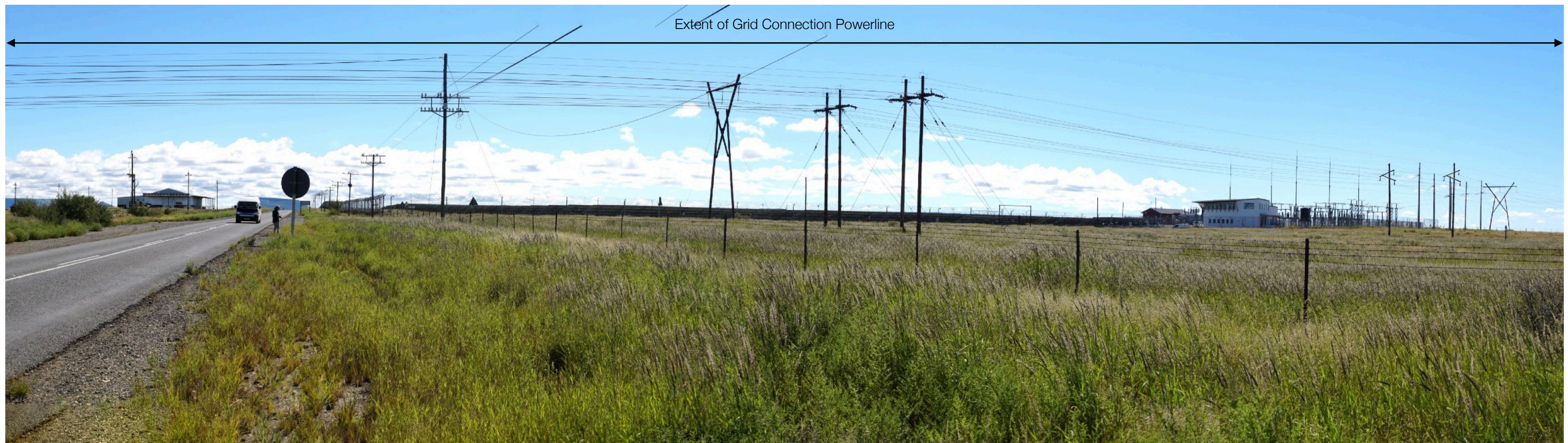
vp3 : Looking North-East from R48 at Grid Connection Crossing
