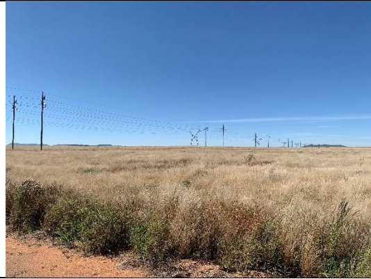
Photo 8: View of the proposed gridline connection route. The proposed route would run parallel to the gridlines in this photograph. This view is in a north-easterly direction.
