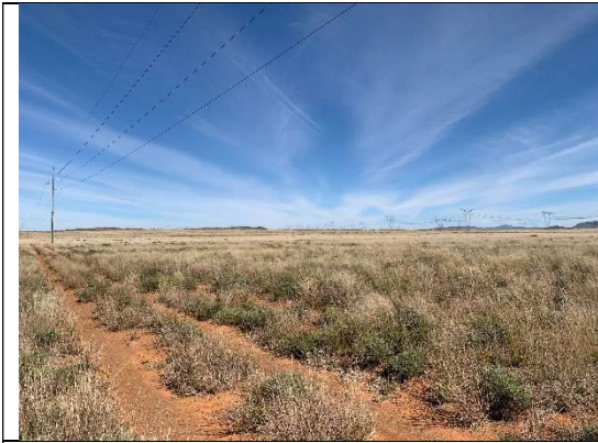
Photo 13: View of the proposed gridline connection route. The proposed line would run in the same corridor of the gridline seen in the foreground of the photograph. This view is in a south-westerly direction.
