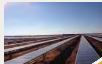
Design, review and site supervision for the Kathu solar photovoltaic (PV) plant
