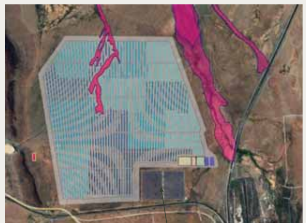
De Aar 10MW solar plant
