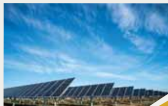
New 132kV Impala Switching Station and 132/11kV, 1x 80MVA Sishen Solar Facility Substation
