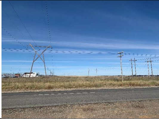
Photo 7: View of the proposed gridline connection from the R43, in an easterly direction. The operational solar facility lies to the north of the proposed route (on the lefthand side of this photograph)
