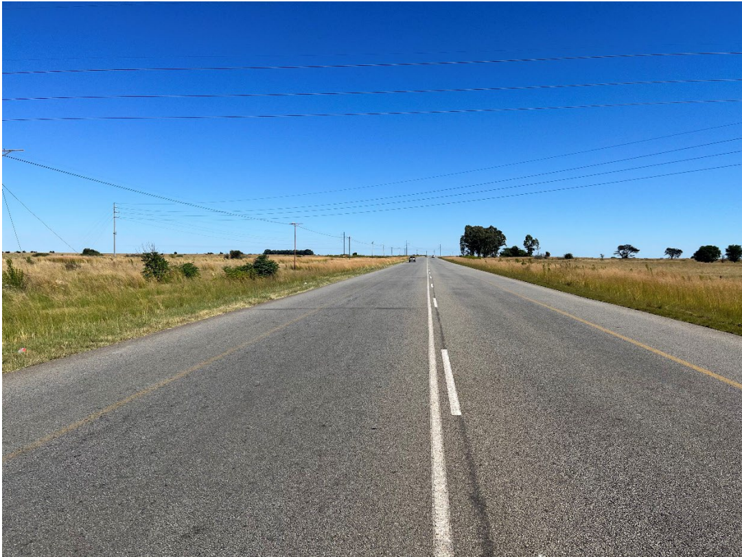
Figure 7.7 Existing Road P28-4 @ Km 7.15 – West Approaching (Access 1)
