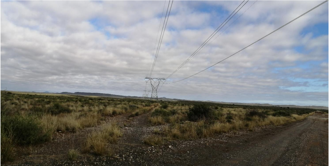
Figure 8: Existing powerlines in the study area
