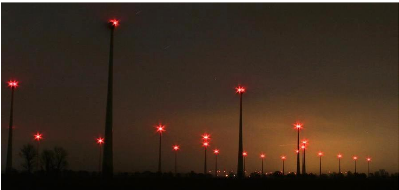
Figure 16: Example of aircraft warning lights fitted to the turbines as prescribed by the CAA 4
