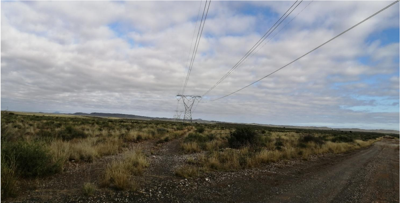
Figure 8: Existing powerlines in the study area
