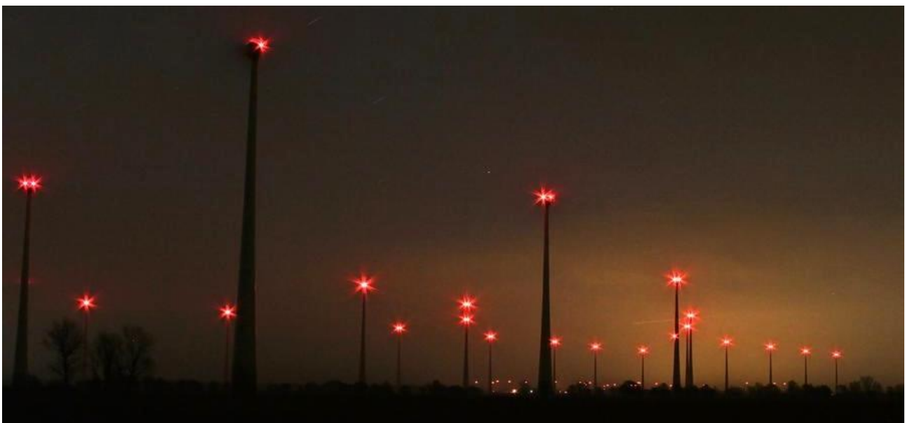
Figure 16: Example of aircraft warning lights fitted to the turbines as prescribed by the CAA 4
