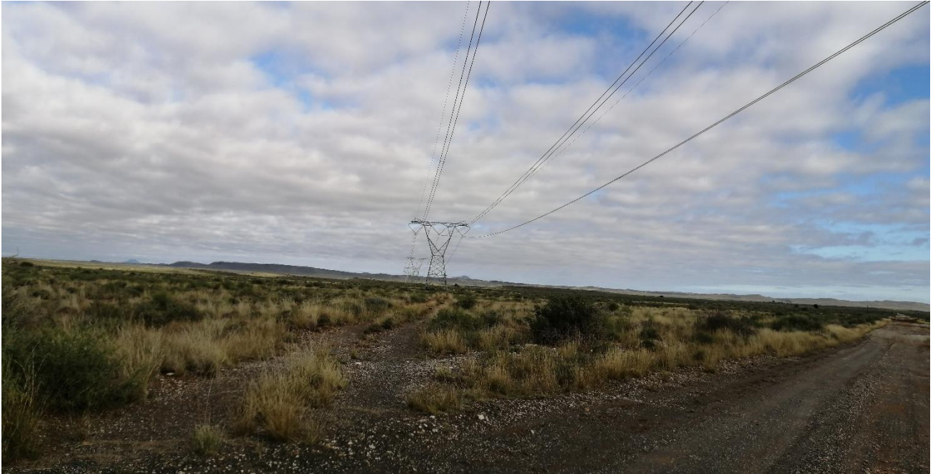
Figure 8: Existing powerlines in the study area
