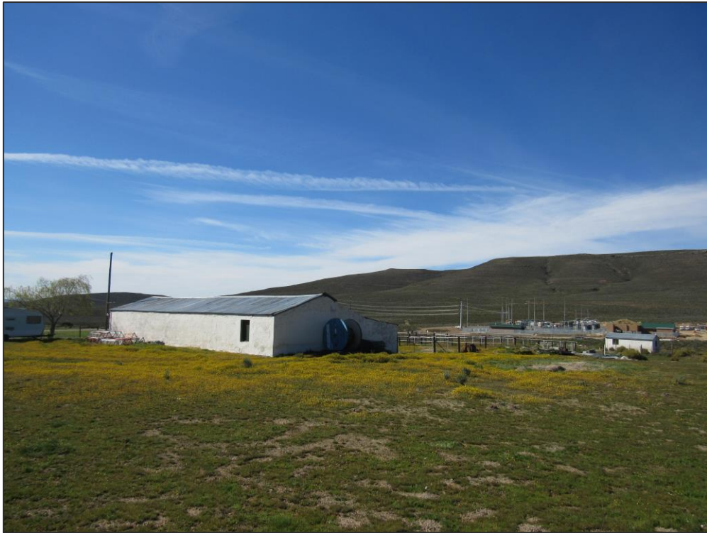
Figure 22: Bon Espirance Substation.
