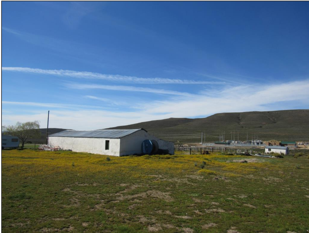
Figure 22: Bon Espirange Substation.
