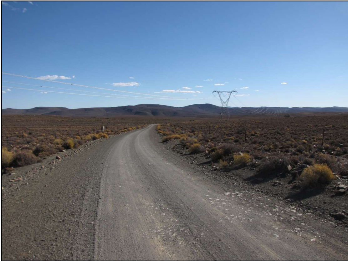
Figure 7: Existing power lines in the study area.
