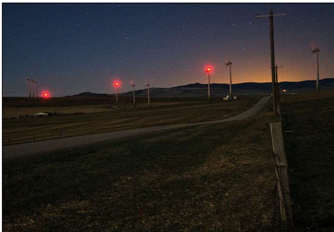
Figure 13: Aircraft warning lights fitted to the wind turbine hubs (Source: http://www.pinchercreekecho.com/2015/04/29/md-of-pincher-creek-takes-on-wind-turbine-lights. )
