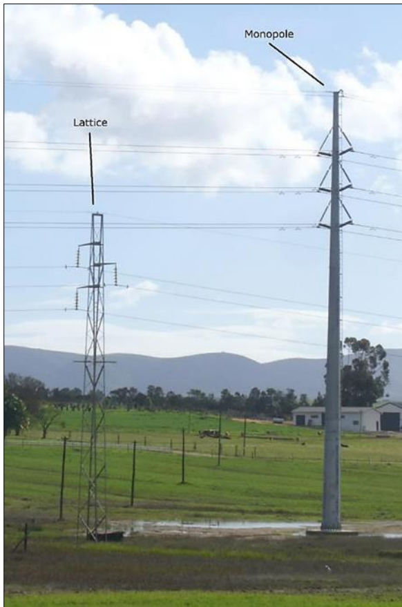
Figure 1-4: Conventional lattice powerline tower compared with a steel monopole structure
