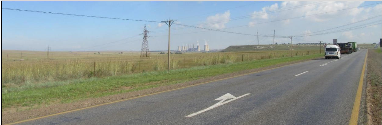
Photograph 3.9: Camden power station and power lines seen from the east from near Mooiplaas colliery on the N2
