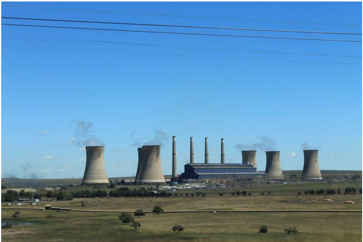
Photograph 3.1: Camden Power Station
