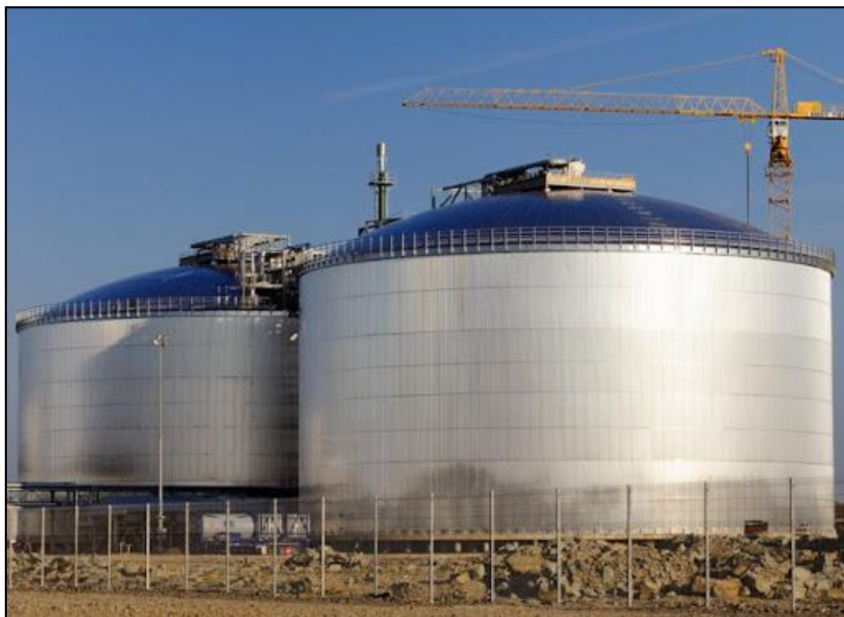
Figure 1.6: Cryogenic ammonia storage tanks
