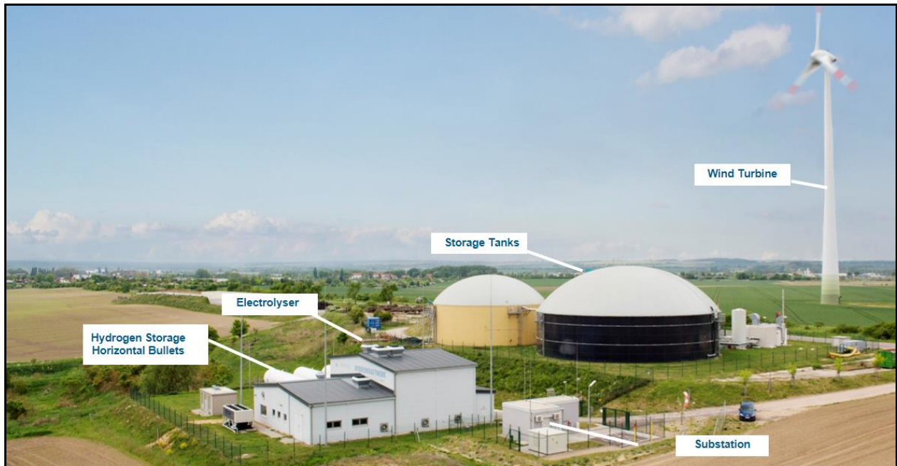
Figure 1.3: Enertrag Hybridkraftwerk Green Hydrogen Facility in Germany
