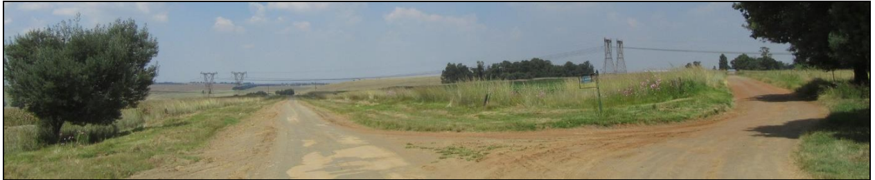
Photograph 3.12: Two 400 kV lines traversing De Emigratie Road
