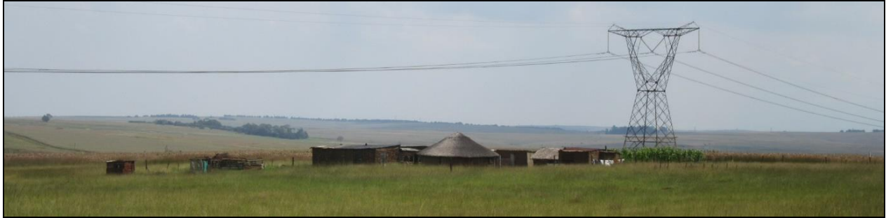
Photograph 3.10: Dwellings of households with tenure rights and 400 kV line on Adrianople farm along the Overvaal road.
