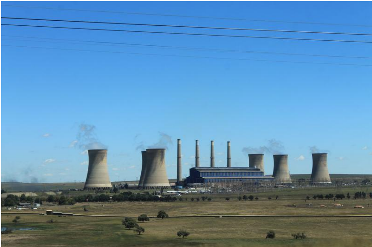
Photograph 3.1: Camden Power Station
