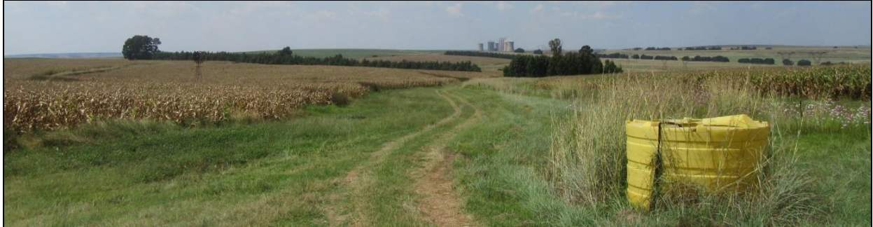
Photograph 3.5: Maize fields on Uitkomst farm along the De Emigratie gravel road with Camden Power station in the background
