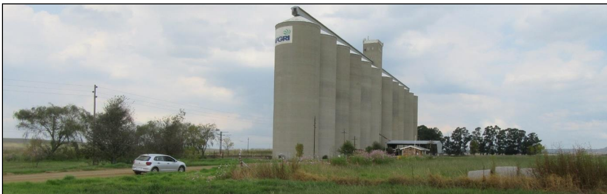
Photograph 3.6: Overvaal silo located adjacent to Richards Bay railway line
