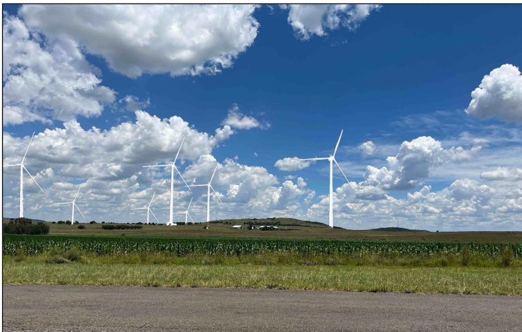
Figure 31: View south-south-west from Losberg Road towards Igolide WEF Project Area (Post-Construction).
