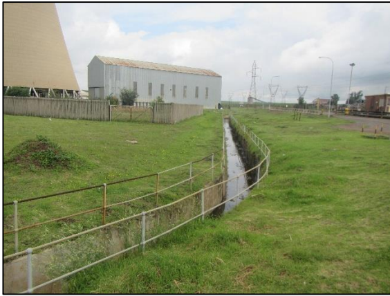
Figure 15: Landscaped lawns adjacent to the Komati cooling towers.
