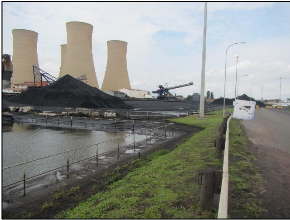
Figure 8: The completely transformed coal deposit area at Komati Power Station.
