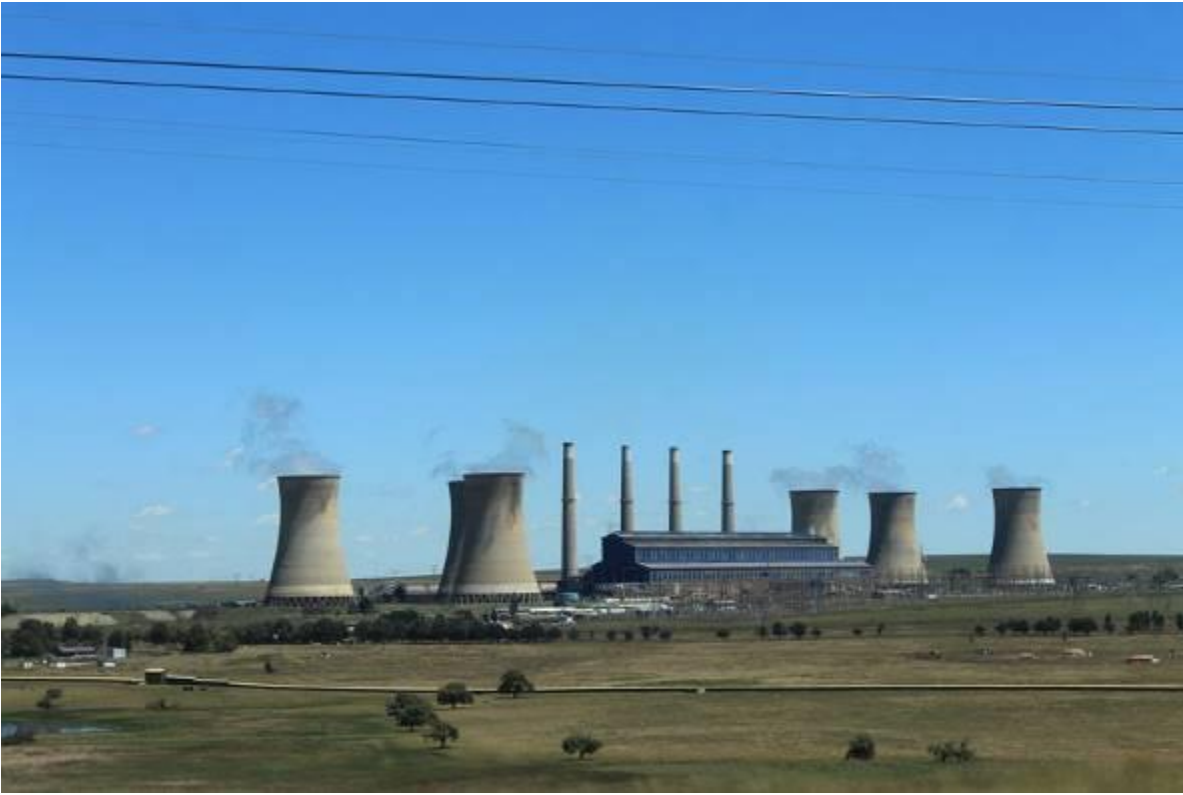
Photograph 3.1: Camden Power Station
