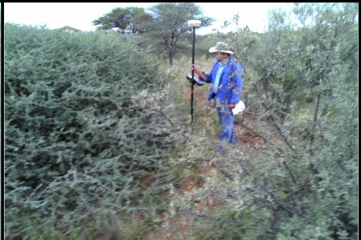
Tower footprint view 2
