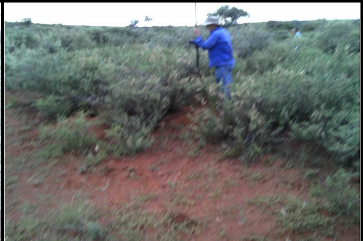
Tower footprint view 2
