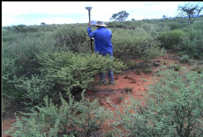
Tower footprint view 1
