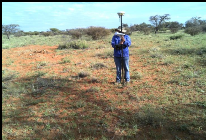
Tower footprint view 1
