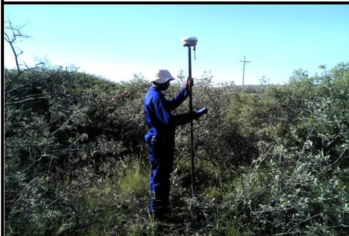
Tower footprint view 1
