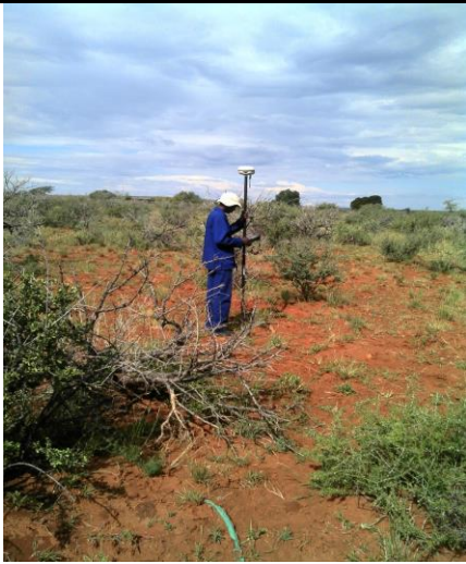
Tower footprint view 1
