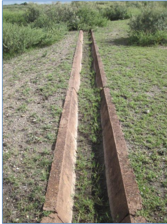
Figure 22 – Concrete furrow
