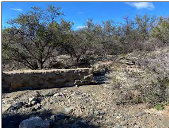
Figure 21: Several small weirs were found within the steeper valleys through-out the study area, most no longer functional
