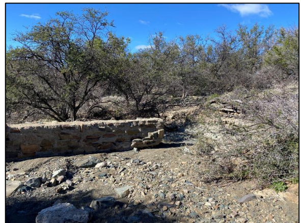
Figure 20: Several small weirs were found within the steeper valleys through-out the study area, most no longer functional
