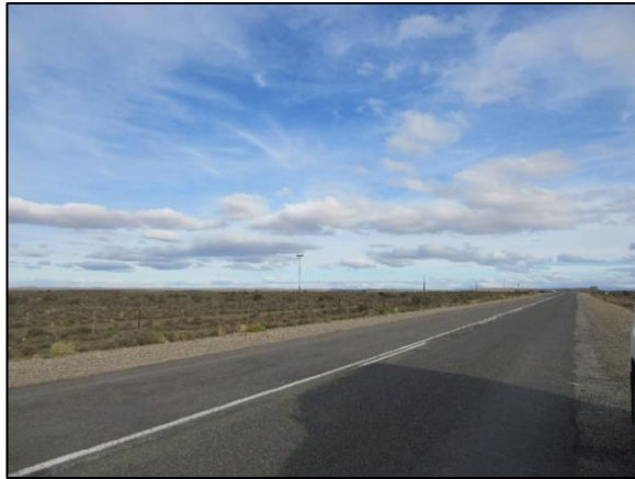
Figure 10: View southwards along the N12 National Route on the eastern boundary of Koup 1 WEF application site.
