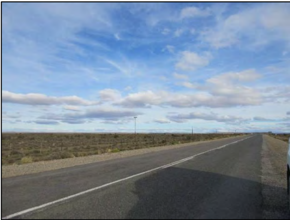
Figure 10: View southwards along the N12 National Route on the eastern boundary of Koup 2 WEF application site.
