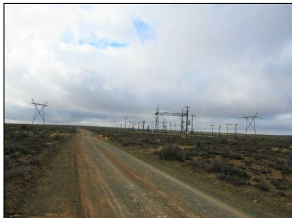
Figure 11: 22kV power lines and associated
