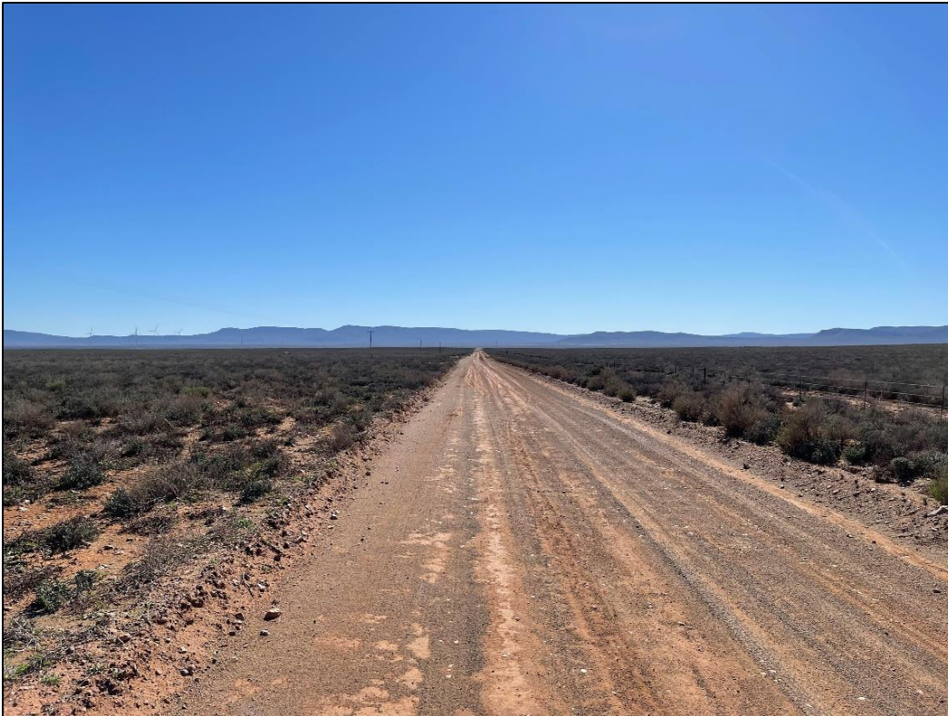
Figure 38: Existing Road OP06121 – North Approaching
