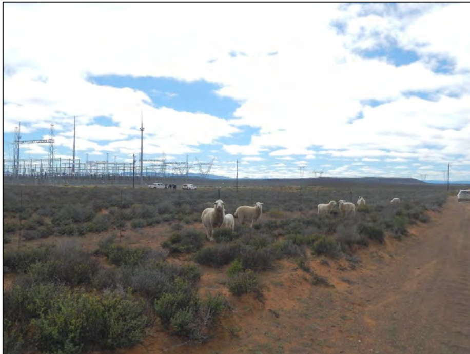
Figure 20: Sheep grazing near Kappa substation
