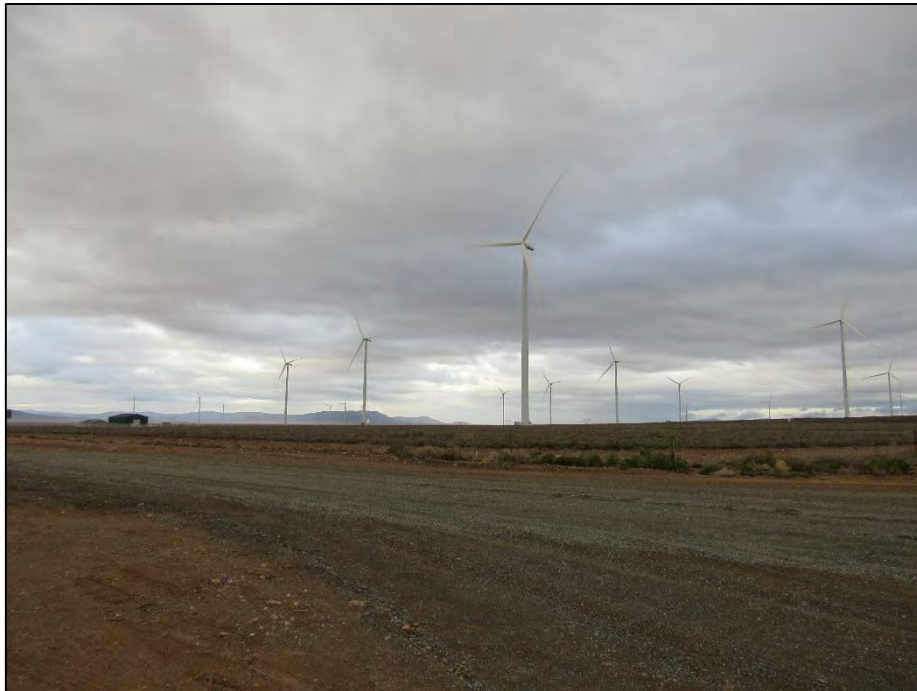
Figure 29: Wind turbines at Perdekraal East Wind Farm, near Touws River, Western Cape Province.
