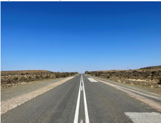
Figure 45: Existing Access to Portion 25 – South Approaching
