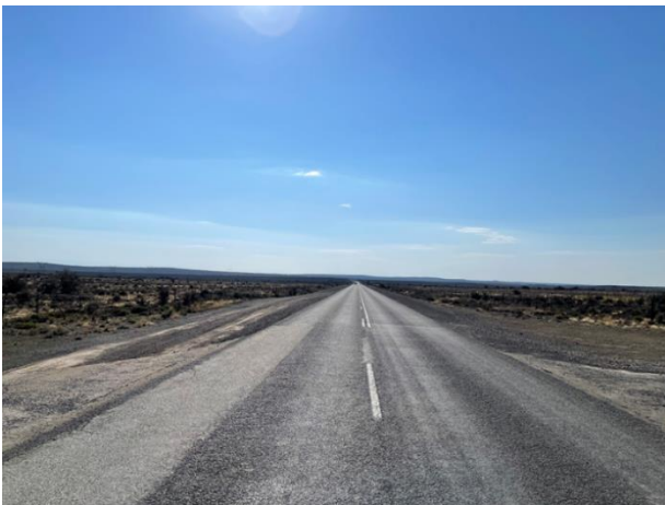
Figure 46: Existing Access to Portion 25 – South Approaching
