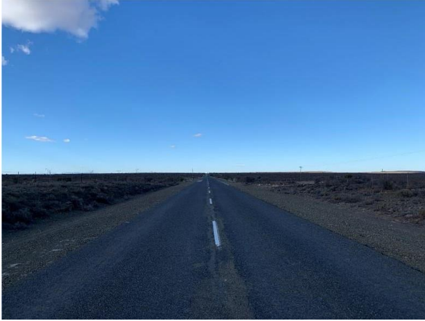
Figure 44: Existing Portion 10 Access – North Approaching
