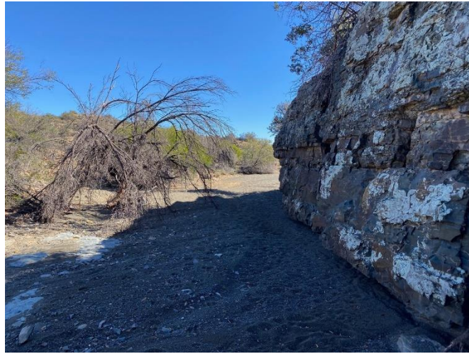
Figure 22: A view of one the few cliffs within the site, that will be avoided by the placement of any turbines, and it's assumed that any of the proposed roads will also avoid any areas with any such slopes
