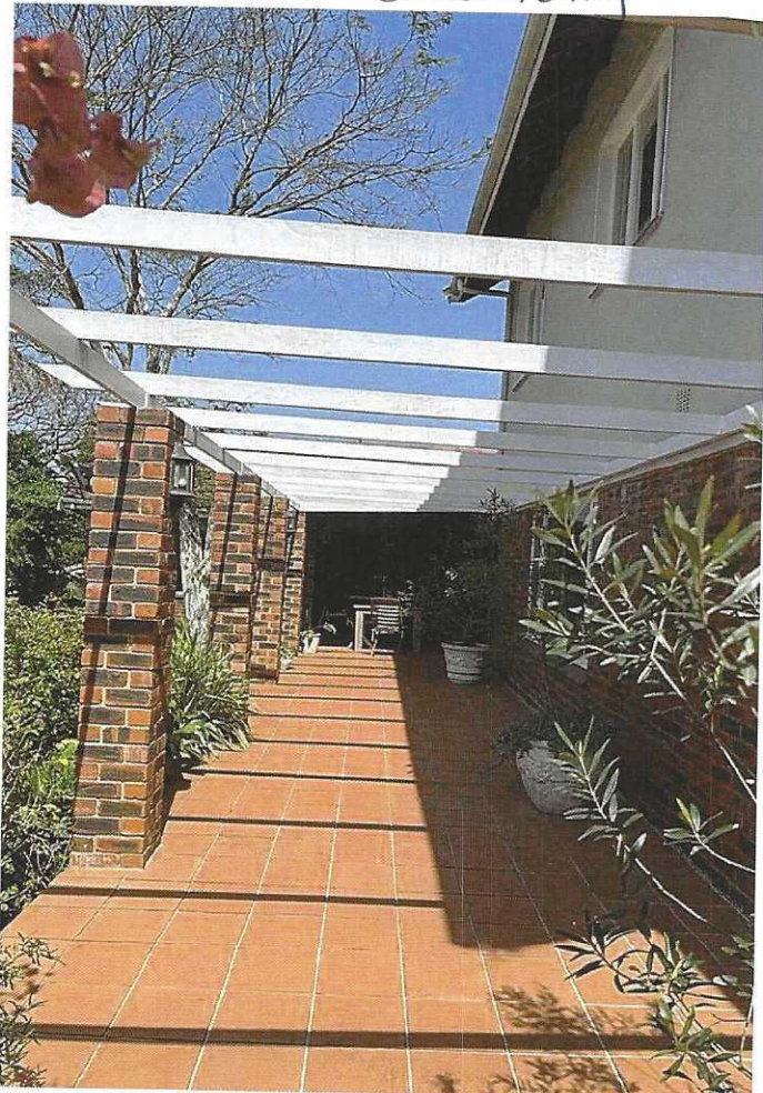
View of existing verandah (S.E.)
