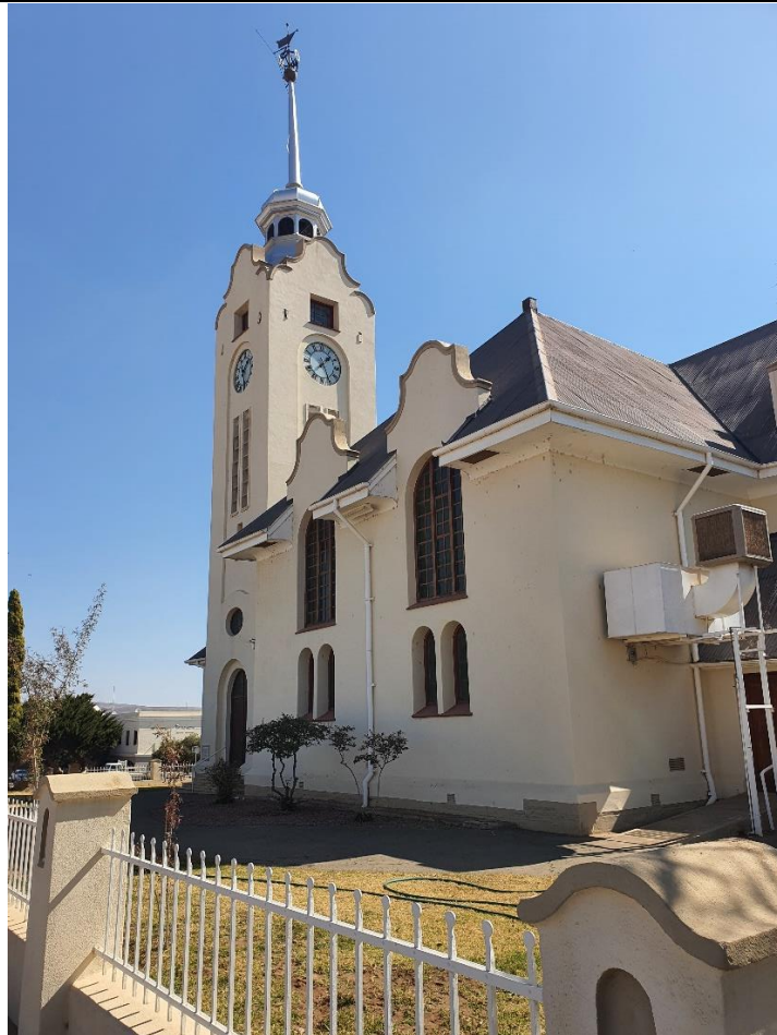
Figure 8: Dutch Reformed Church situated within the CBD of Prieska.
