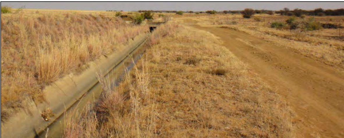
Figure 7-25: Sand-Vet Irrigation Scheme concrete canals traverse the project area
