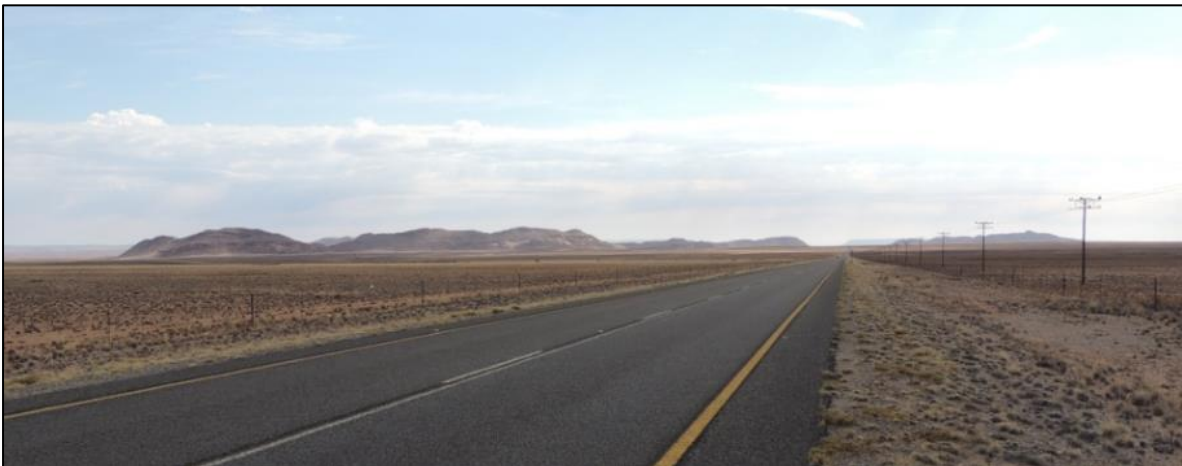
Figure 10: N14 National Road northbound just before Aggeneys Town
