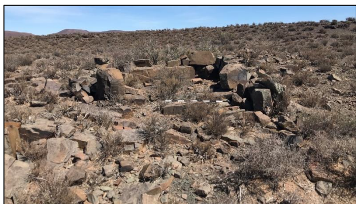
Figure 31: K-08 Collapsed stone shepherd's shelter
