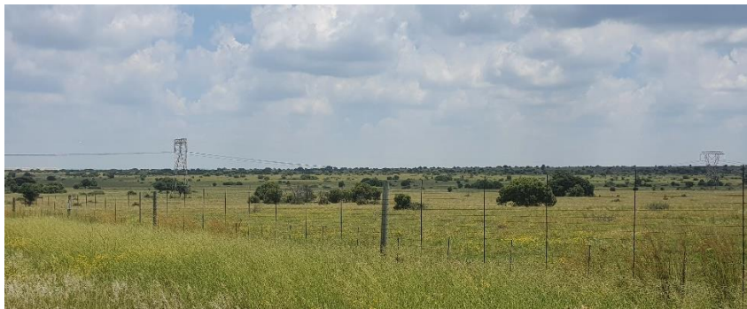
Figure 4-4: Hermes/Pluto 400 kV powerline
