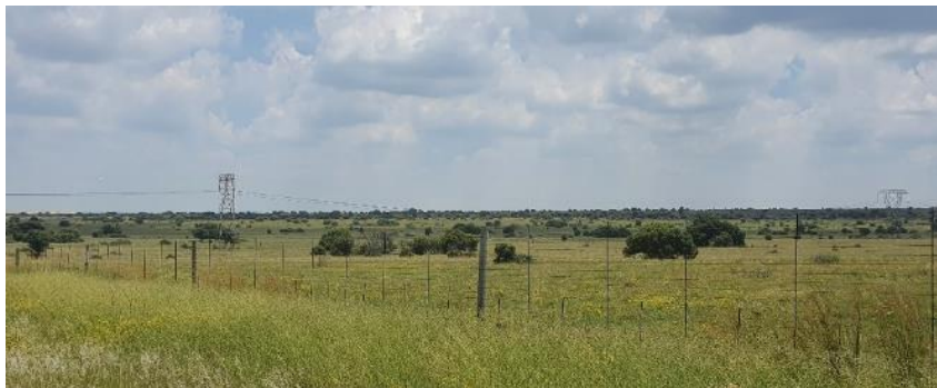
Figure 4-4: Hermes/Pluto 400 kV powerline
