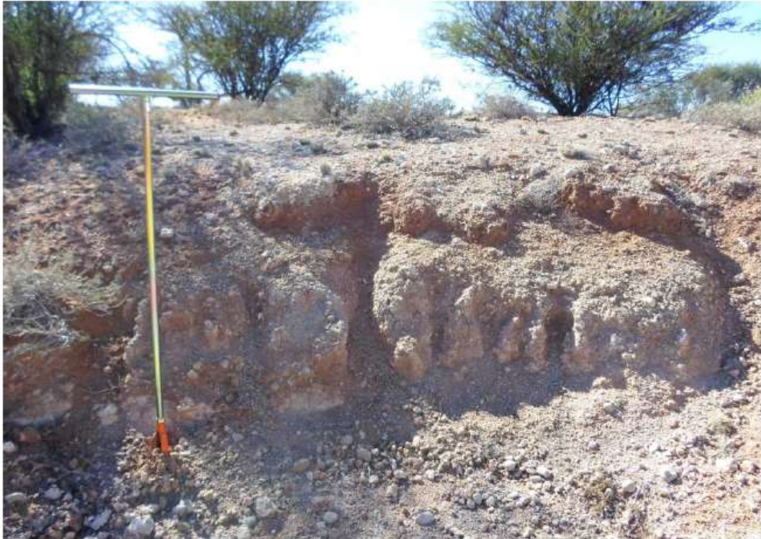
Figure 3-7 Eroded ephemeral drainage line embankment with weak soil structure containing a low clay percentage (Savannah Environmental, Draft 2015)
