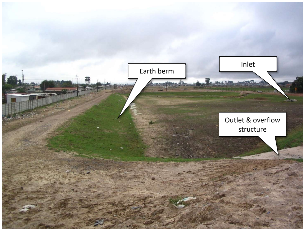
Figure 3-4: Detention Pond Example
