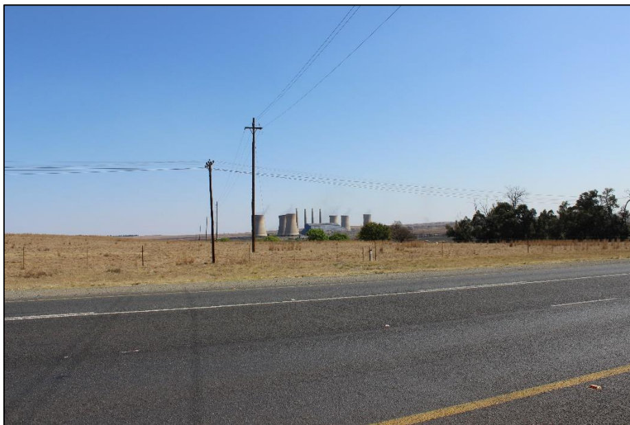
Figure 16: View of Camden Power Station to the west of the N2 national route.
