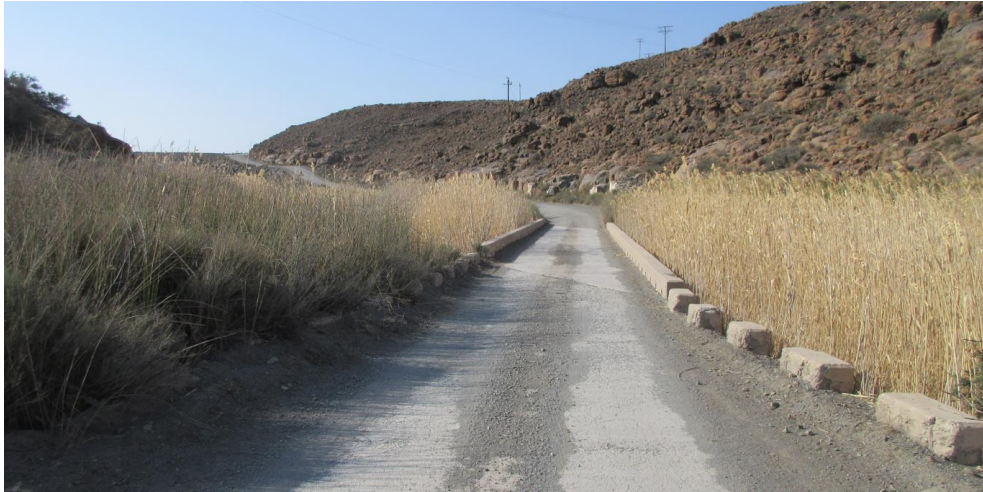
Figure 8 - Narrow Single Lane Low-Level Bridge
