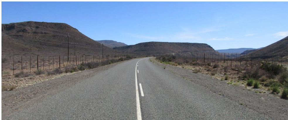
Figure 6 - TR05801 - Paved Section
