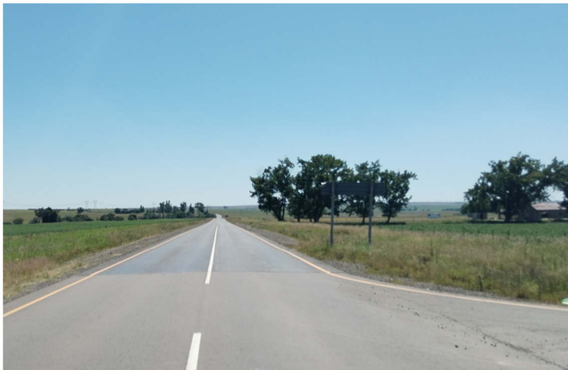
Figure 4-8: Sight distances from access point 2 in a north-eastern direction
