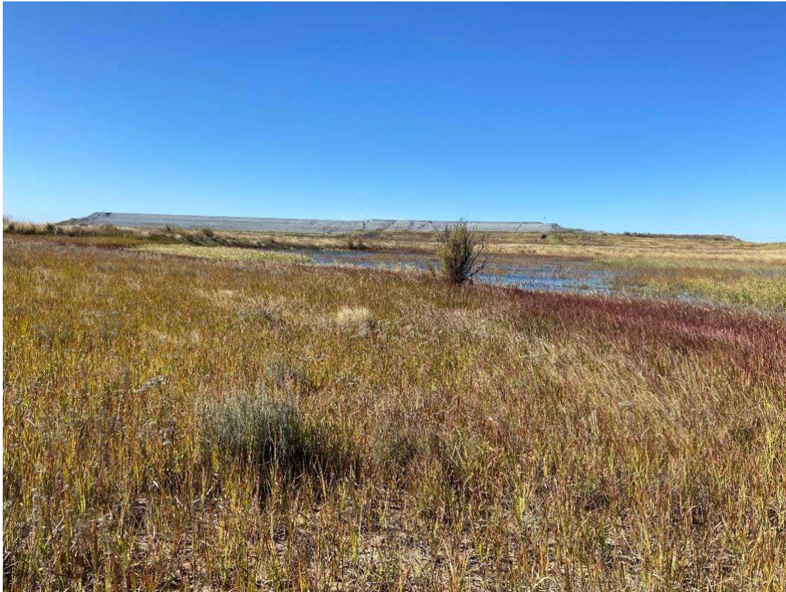
Figure 5-13 - Ash dam facility and pooling of water at dam
