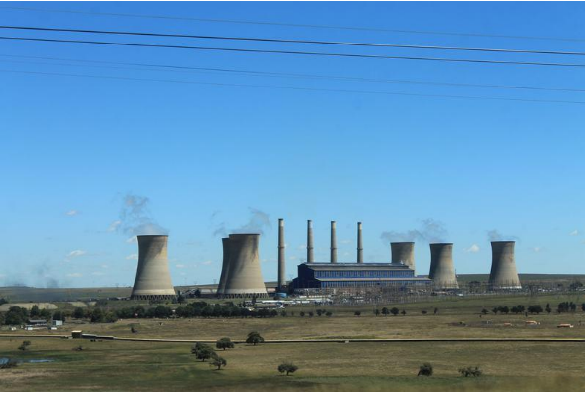
Photograph 3.1: Camden Power Station
