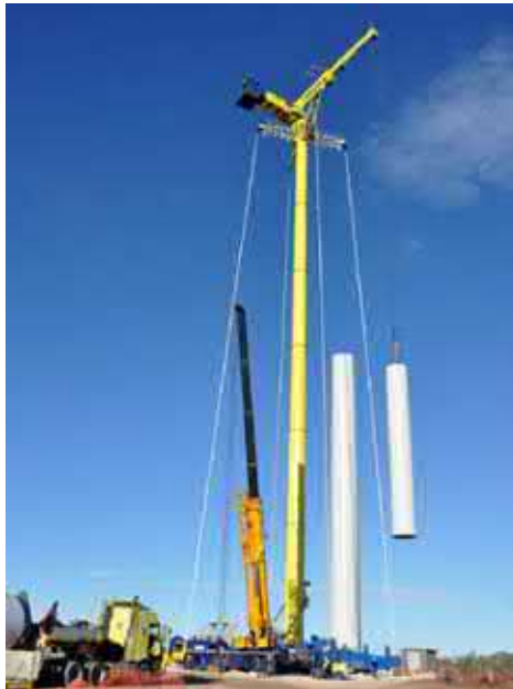
Figure 4-6: Cranes at work
