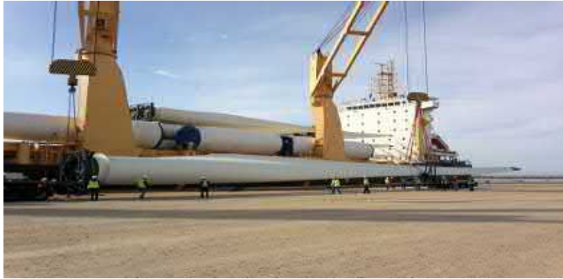
Figure 4-7: Cranes at Port of Entry
