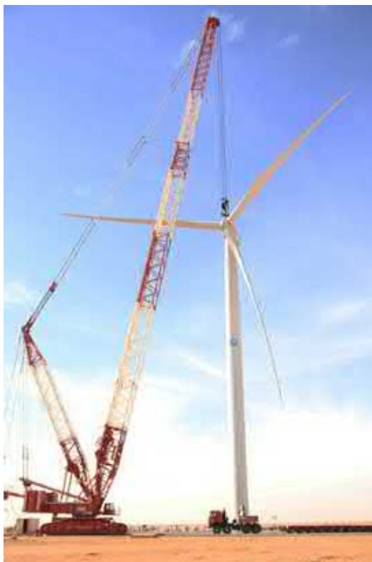
Figure 4-5: Crawler Crane used to assemble turbine (Liebherr, 2017)
